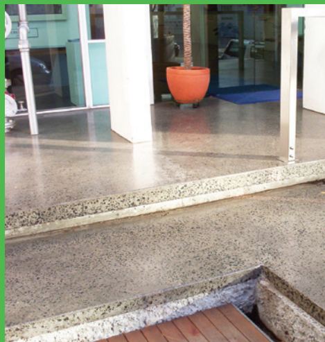
Deep grind - hone and urethane seal
