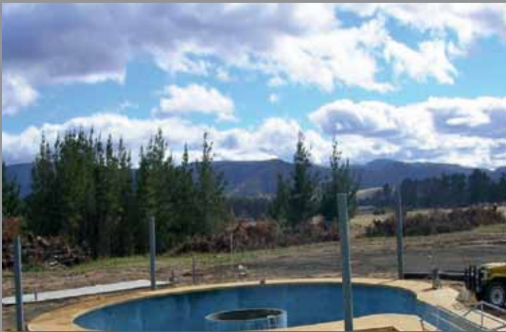
Active crystal growth waterproof liner to horse training pool. Colour, impact, abrasion resistant
