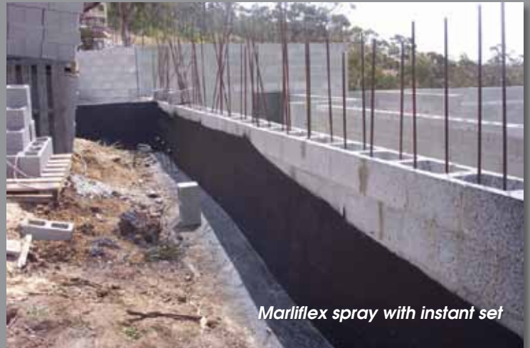
Full system installation Marliflex, Atlantis Drainage panel, Geofabric with soil and grass over. Hobart University Students Union
