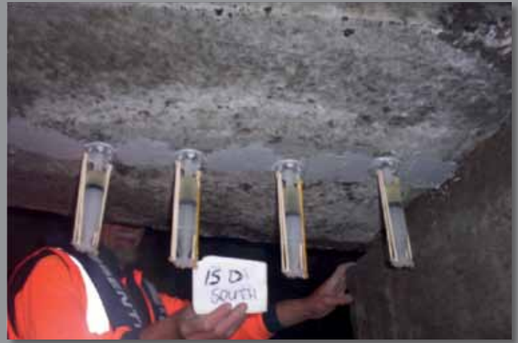
Crack injection of epoxy reconsolidate concrete substrate before applying membranes or coatings
