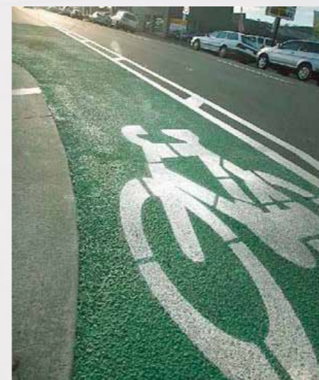
Left: Two Colour Coats encapsulating anti-slip granules to cyclist safety areas.
