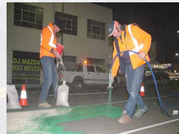
Left: Two Colour Coats encapsulating anti-slip granules to cyclist safety areas.
