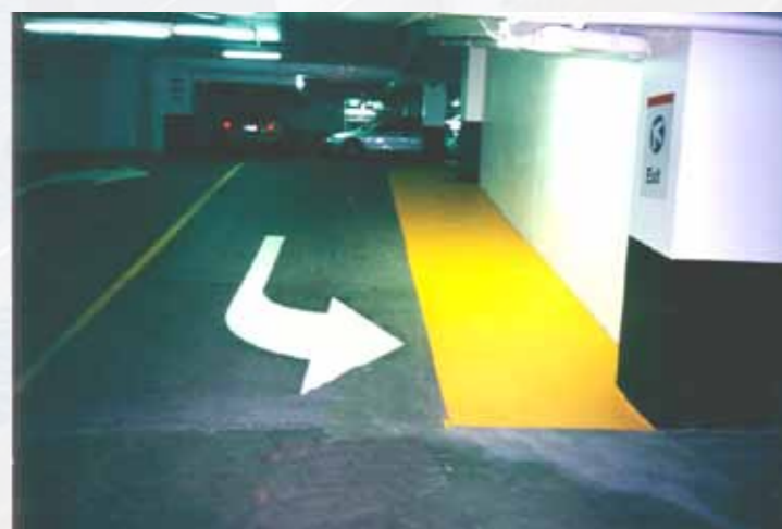
TT Line access ramp & deck sections Degaroute coating
