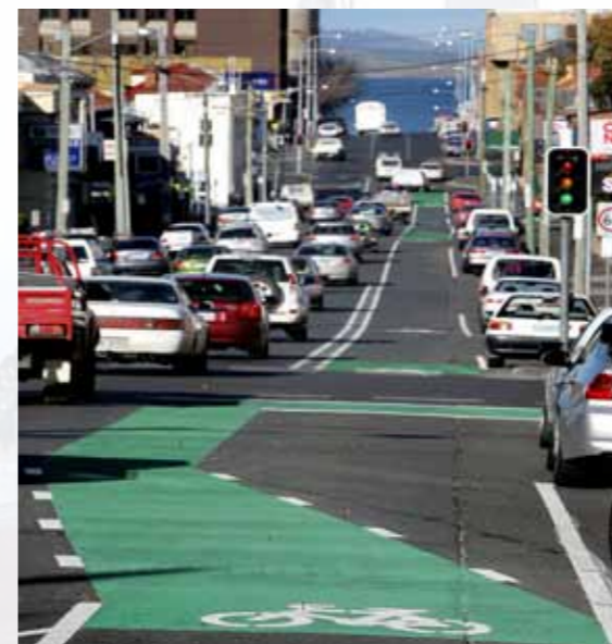
Hobart's cycle lanes installed by Maintenance Systems in Argyle & Campbell Streets.
