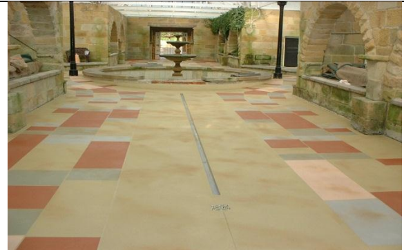
Blocked multi colour spraypave sandstone look
